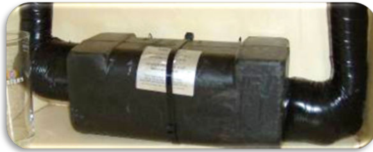
Example of correctly insulated pod
